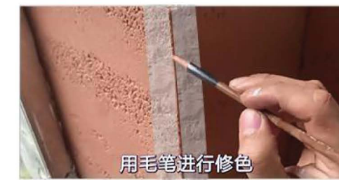
11.用修色剂进行修色 Use a color modifier to repair the surface color
