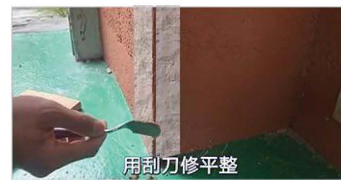
9.用刮刀修平整填缝剂 Use a scraper to smooth the caulk
