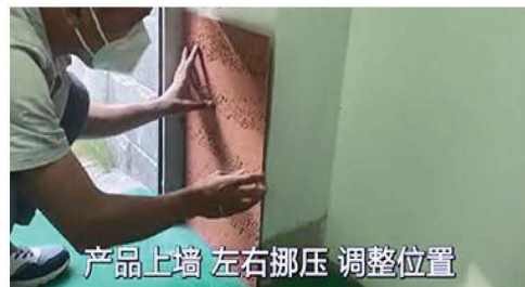
2.产品背后打胶上墙 Glue the back of the product onto the wall
