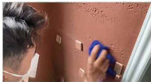
5.铺贴后使用干布清洁 Clean it with a dry cloth after paving
