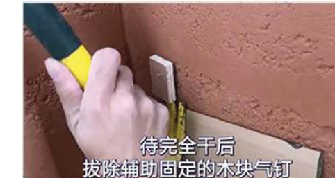
12.待完全干后拔出气钉 After it is completely dry, pull out the air nails
