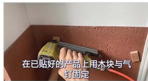
3.用气钉固定 Fit it with air nails
