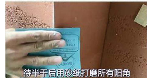
10.打磨 Grind the edges and corners
